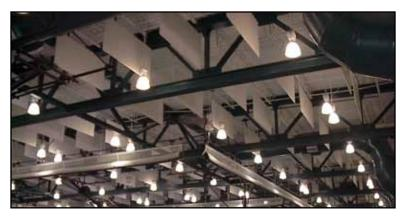
Sound Control Baffle | Model KB-803 Available in FDA and USDA approved construction for food processing industry. Standard fiberglass absorbers are faced with a heat sealed white or black fire retardant vinyl and equipped with two grommets for hanging. Meets Class 1.
