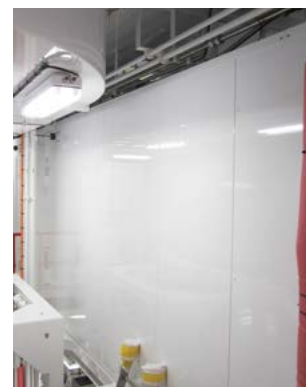
Sound insulating walls for engine room
