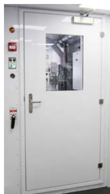
Sound insulating doors and windows for engine room
